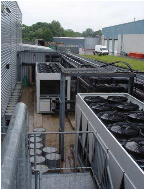
DeltaChill™ FreeCool chillers providing free-cooling to indoor units in a Manchester data centre
